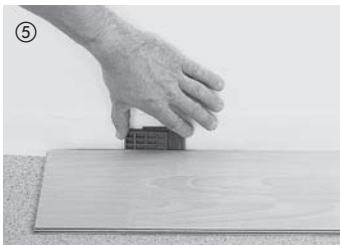
Starting in the right-hand corner of the room, align the boards of the first row with the tongue side parallel to the wall, and fix them in place with wall spacers as you proceed (always keep an expansion gap of 10–15 mm around perimeter).
