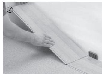
Cut the last board of the first row to size, leaving an expansion gap of 10–15 mm between the board and wall. Insert the board at a slight angle and rotate it down. Start the second row with the leftover piece of the first row (offset the end joints of adjoining rows by at least 40 cm). This considerably reduces waste.
