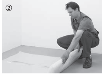
Always use 0.2 mm thick PE film overlapped by 30 cm as an underlay when laying your floor over all types of floor screed. The overlap seams must overlap by 30 cm. Extend underlay up all walls. After having installed the skirtings cut underlay at the upper edge of the skirtings.
