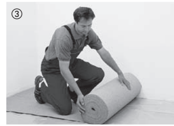
For sound insulation and to smooth out slight irregularities of the subfloor, unroll 2 mm thick cork underlay. Do not overlap. Our range of accessories also offers alternative insulation underlays. Asphalt-bitumen felt is not suitable for sound insulation. Do not use any additional insulation underlay when laying HARO laminate floor with Silent Pro®.
